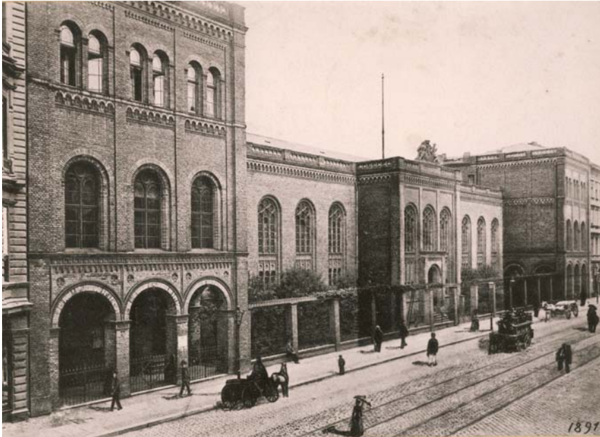
FIGURE 14 Municipal gymnasium in Berlin Prinzenstraße, converted into a hospital during World War I
